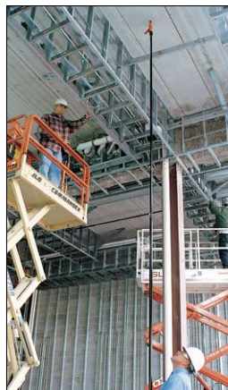
The Viper screws solidly onto a pole for high reach and secure operation for ceiling applications.
